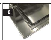
Check the door seal and ensure it is intact, not hanging loose or any sections broken away. Report defects and advise on replacement as required SA3113.
